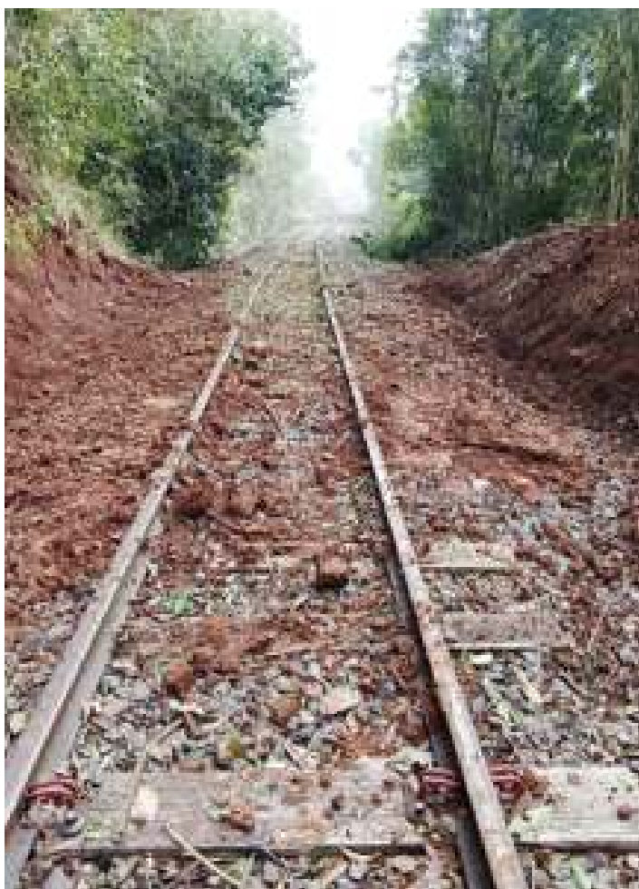
♦ Limpeza barreira km 855+600.
